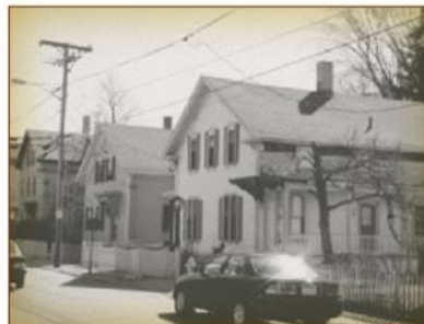
These tidy Greek-Revival houses from the 1840s are just one example of the mill worker housing that still exists in the South Central Falls Historic District.
