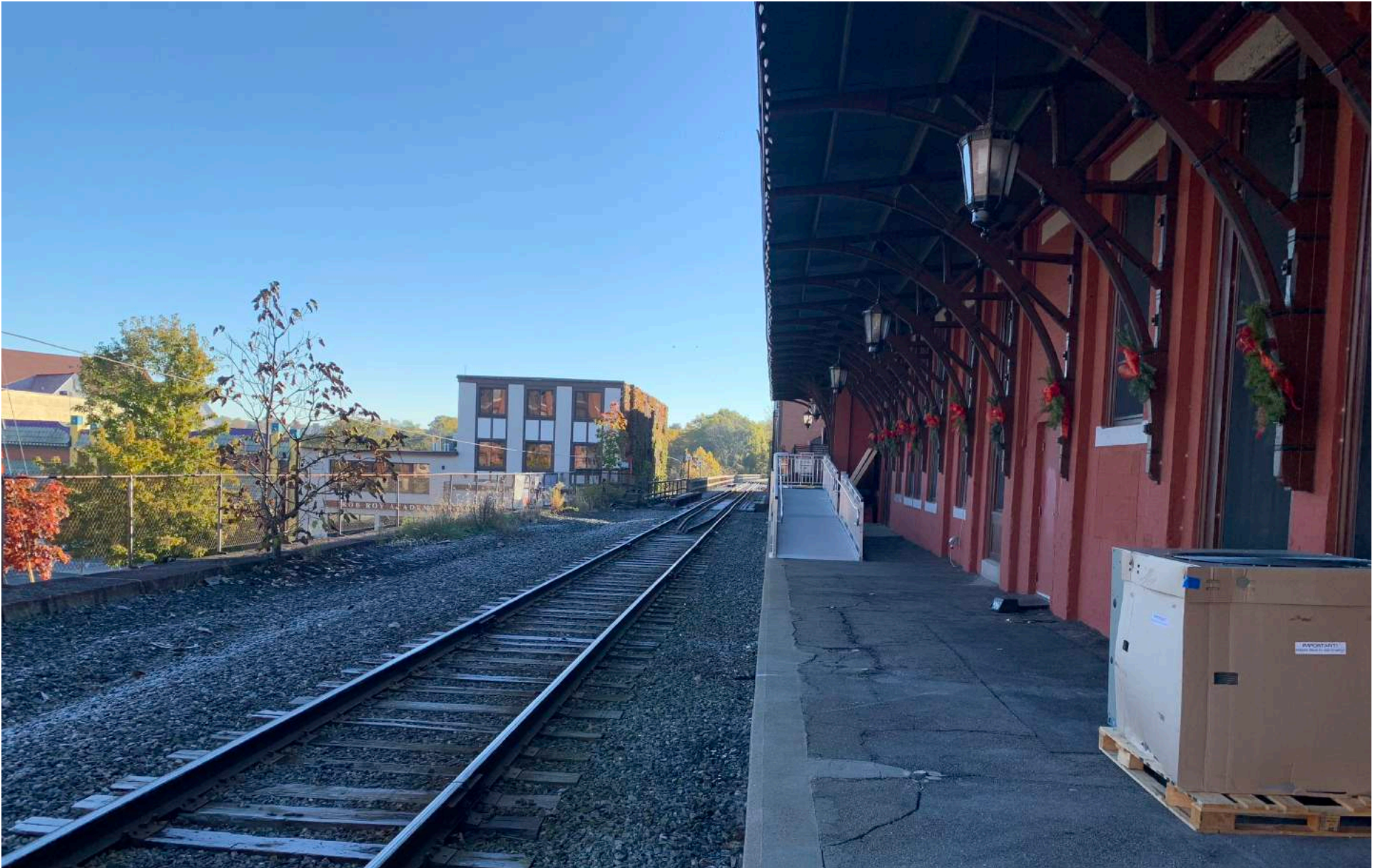
Figure: Photograph of Polar Express Station Platform. Source: Report authors.
