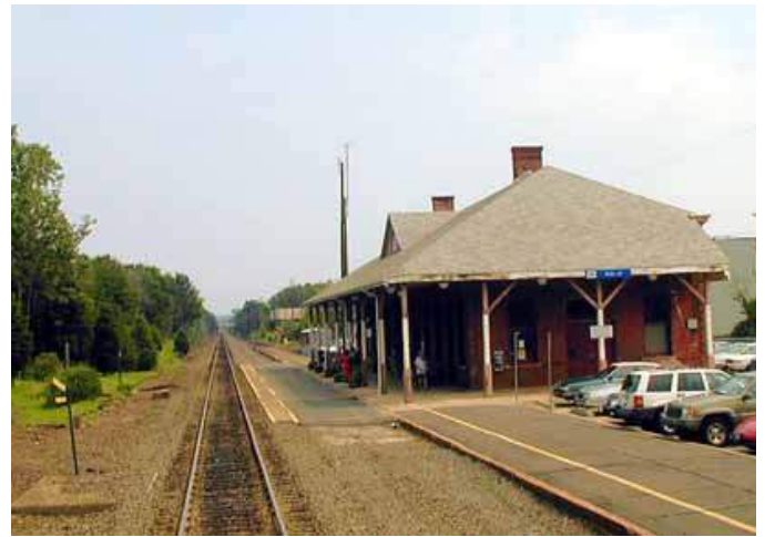
Figure: Old station remains and new platform construction at Berlin, CT station. Source https://commons.wikimedia.org
